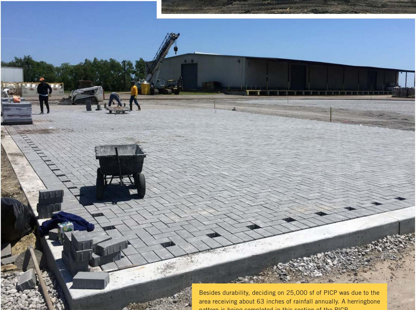
Besides durability, deciding on 25,000 sf of PICP was due to the area receiving about 63 inches of rainfall annually. A herringbone pattern is being completed in this section of the PICP.
