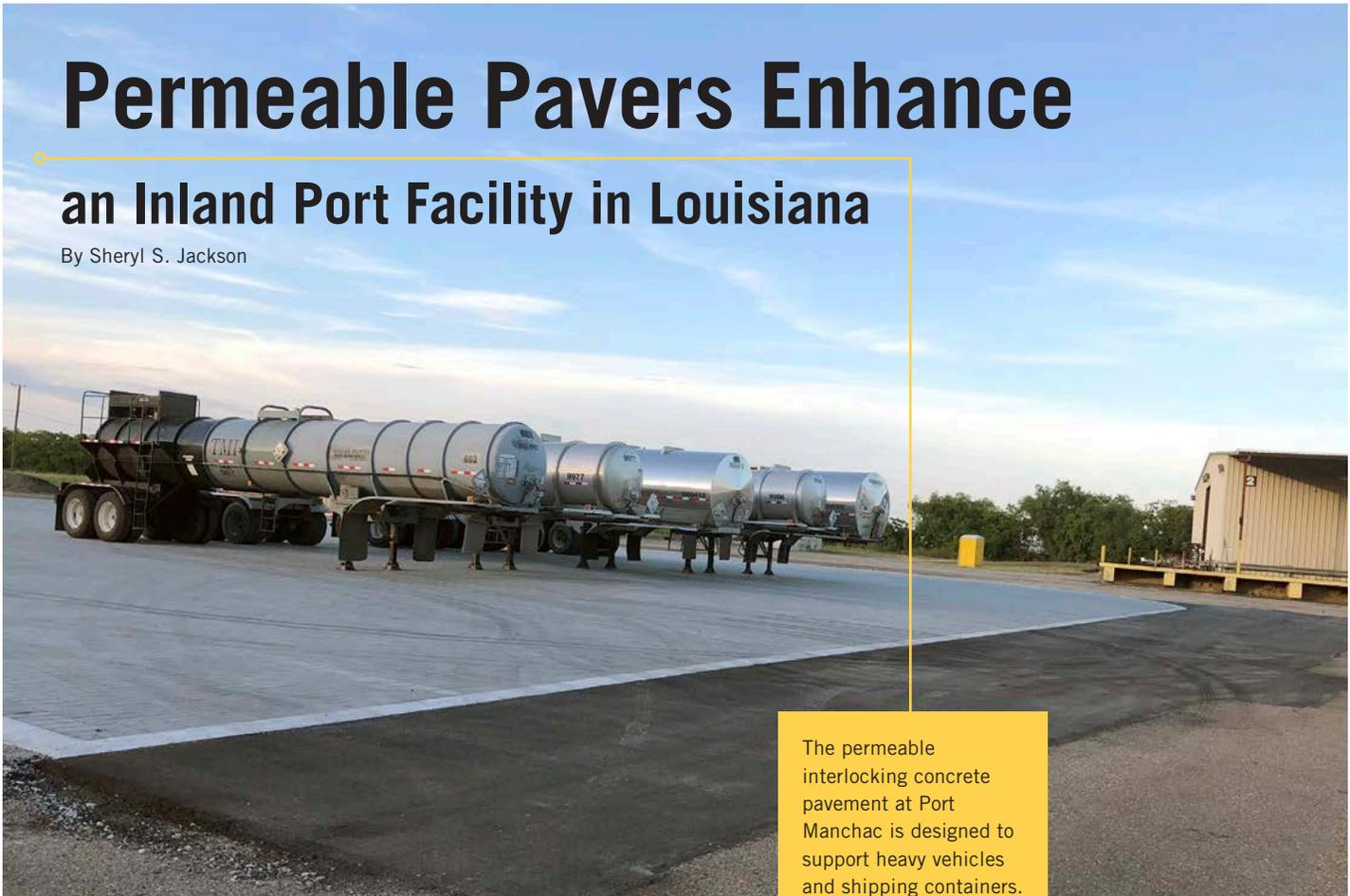
The permeable interlocking concrete pavement at Port Manchac is designed to support heavy vehicles and shipping containers.
