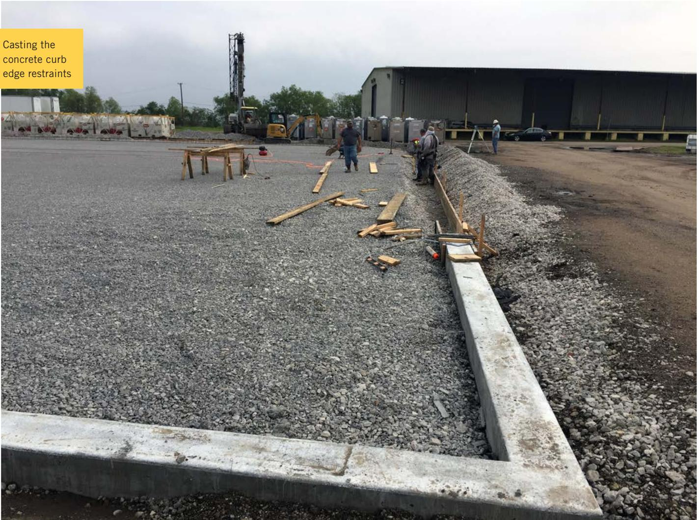
residential applications,” he explains. “I was a little apprehensive about an open-graded subbase and base supporting a permeable paver system under the port traffic, but it is working well,” he admits.
